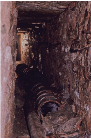
Figure 2 The gallery with terracotta and iron pipelines (by Metin Albukrek)
