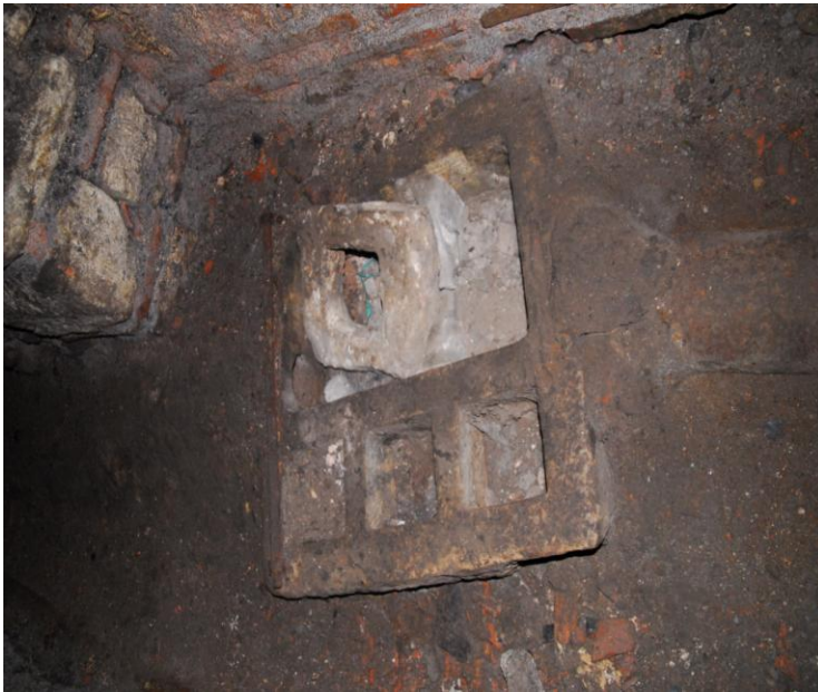
Figures 9 & 10 The Water Distribution Chest under Sphendone and its Drawing (by Çiğdem Aygün – Drawing by Atilla Bir and Mustafa Kaçan)
